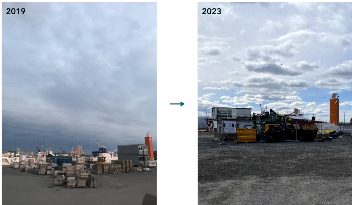
Photo 10 & 11: Construction at Sukkerbiten over the years (Thea Wikander 2019, 2023).
