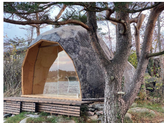
Third tarring with charcoal and shell sand April 2021. Mounting of the glass Oct. 2021
