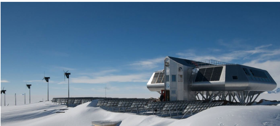
Figure 1. PV plant affected by snowdrift development at the Princess Elizabeth station in Queen Maud Land, Antarctica. (SMA Solar Technology AG, 2019).
