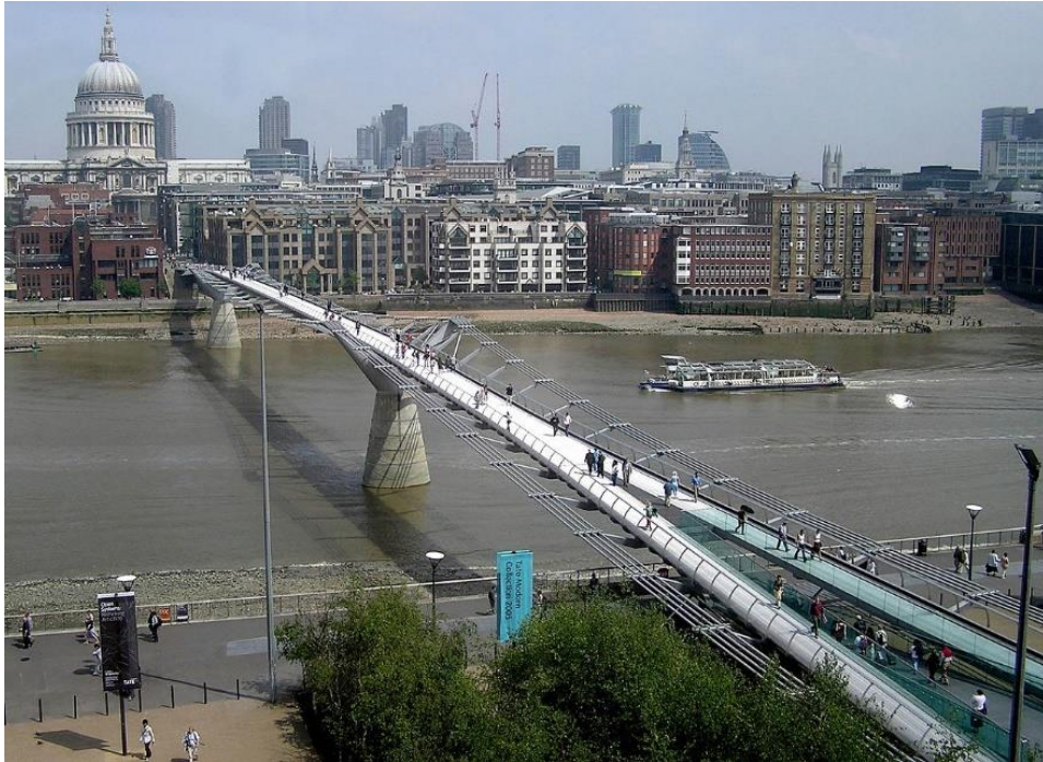
Figure 1.1: The London Millennium Bridge
