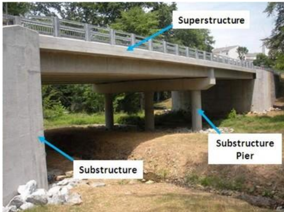
Figure 2.5: the figure illustrates the placement of the different structures described above. The figure is extracted from Hartford County (Miller, u.d.)
