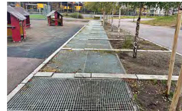
Vannrenne under rist
