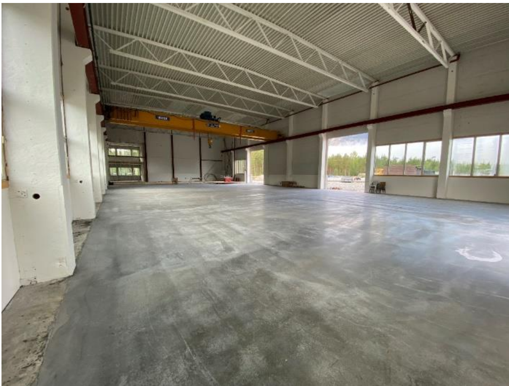
Figur 16: Betongsøylene i Fyresdal fabrikkhall. Foto: Resirqel AS
