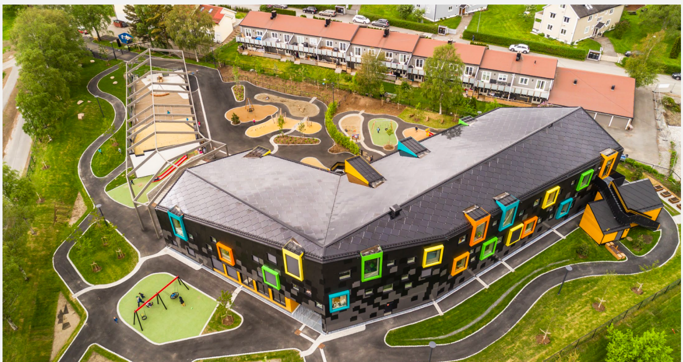
Figure 2 Kilden kindergarten, overview
