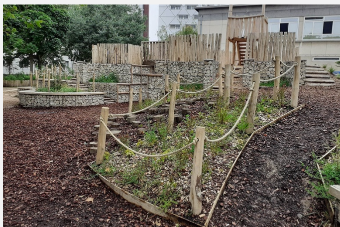
Figure 32 Gabions and rain gardens forming a playscape
