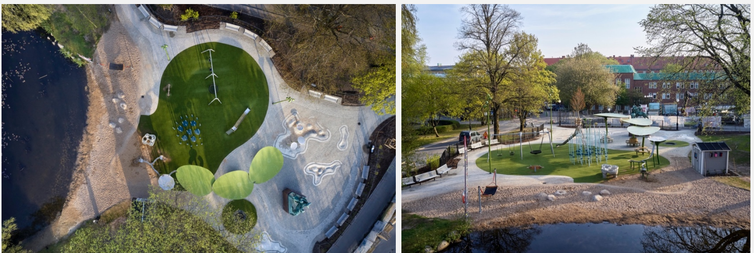
Figure 24 Plan view of the rain playground and the recreational space around it
