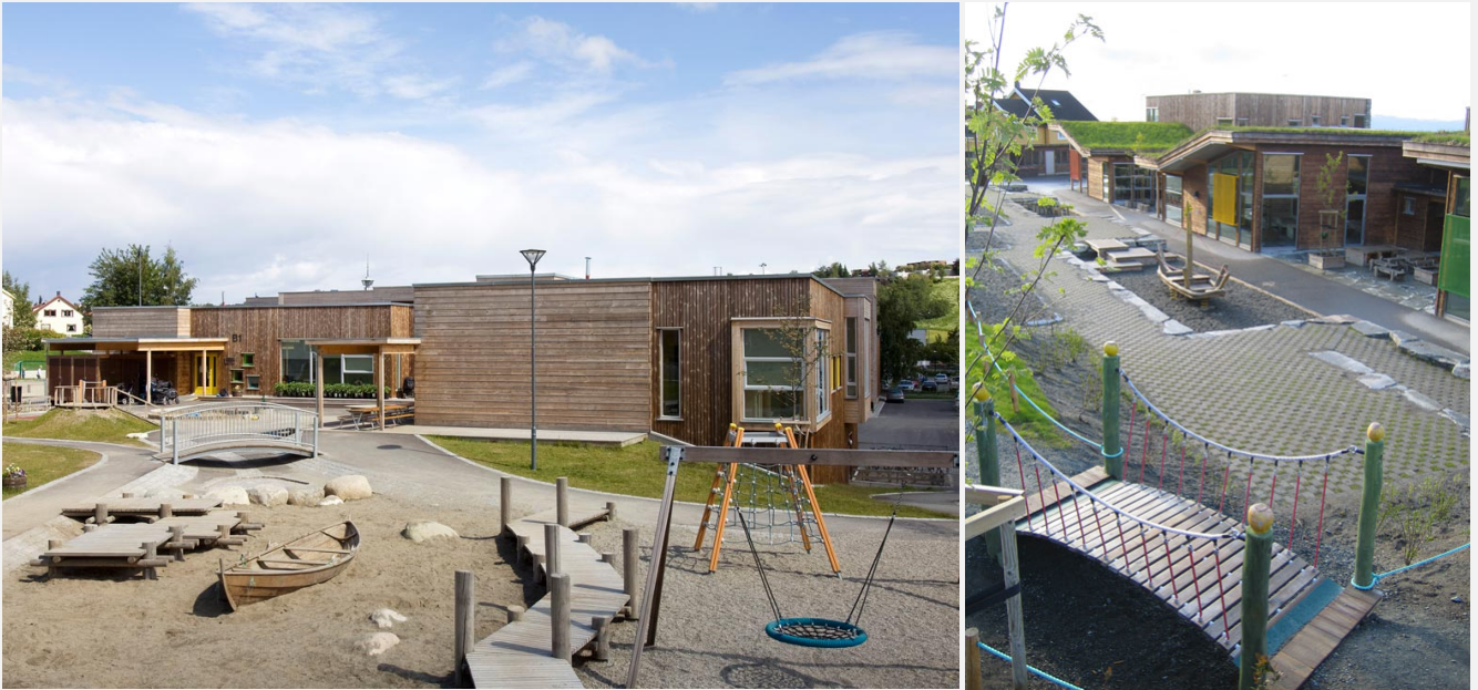
Figure 30 Sand and permeable surfaces at Nardo and Solbakken kindergartens, Trondheim
