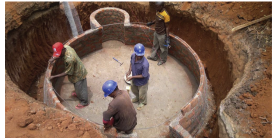
Fig. 3. Bio-digester under construction: Meskan District, Southern Ethiopia (SNV [65]).
