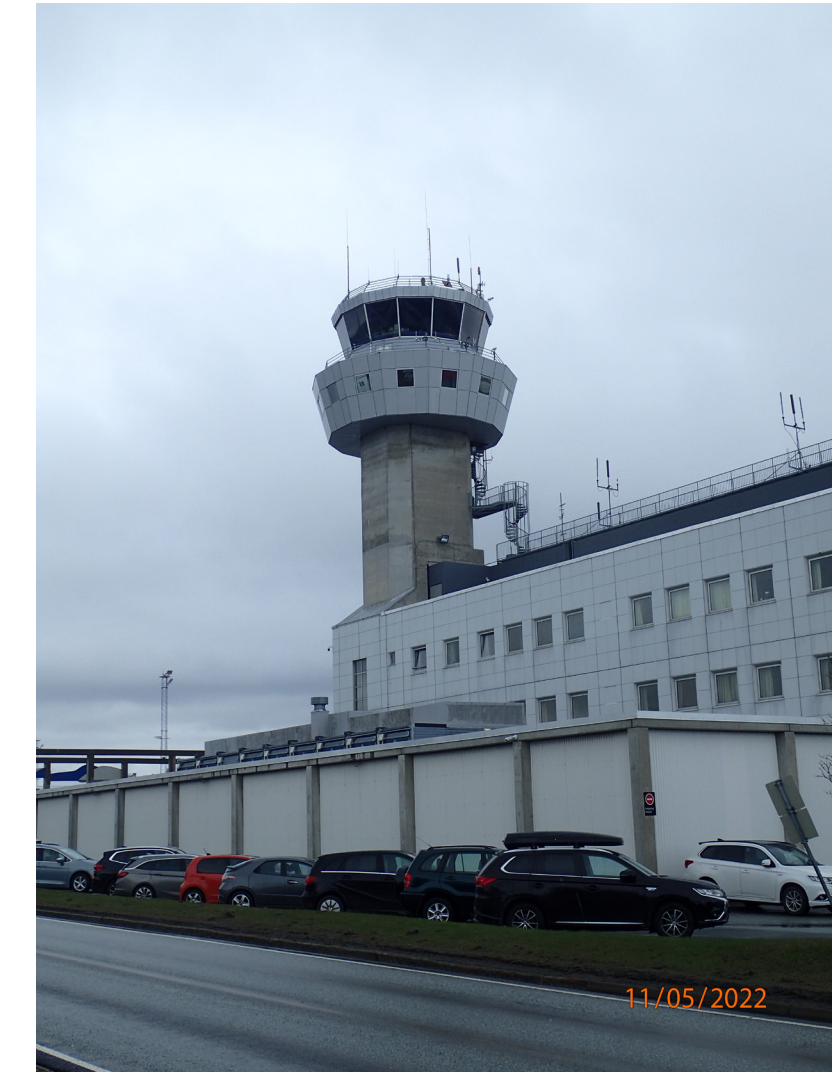
Figure 31. The air traffic control tower seen from Olav 5 gate. Bodø, 11 May, 2022.
