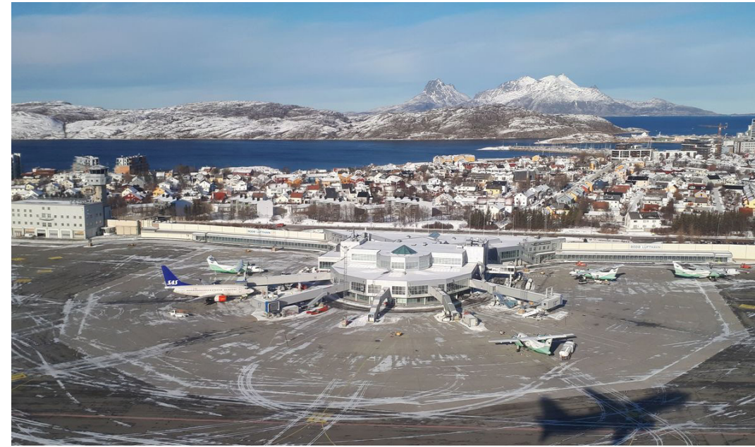
Figure 27. The terminall hall seen from the southern side, n.d, (Photo: Engerengen, L.).
