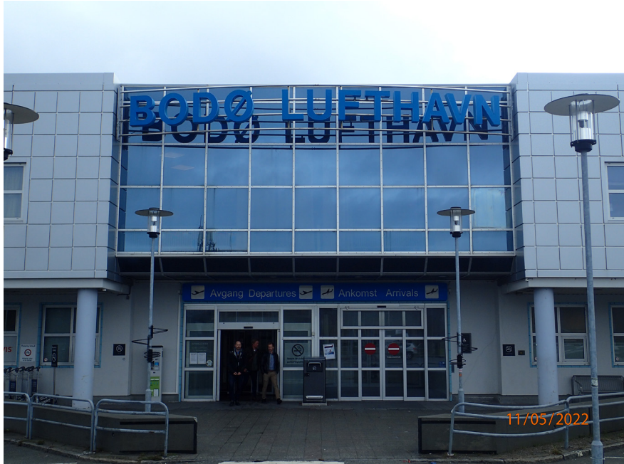
Figure 70. Outside the main entrance of the terminal building. Bodø, 11 May, 2022.
