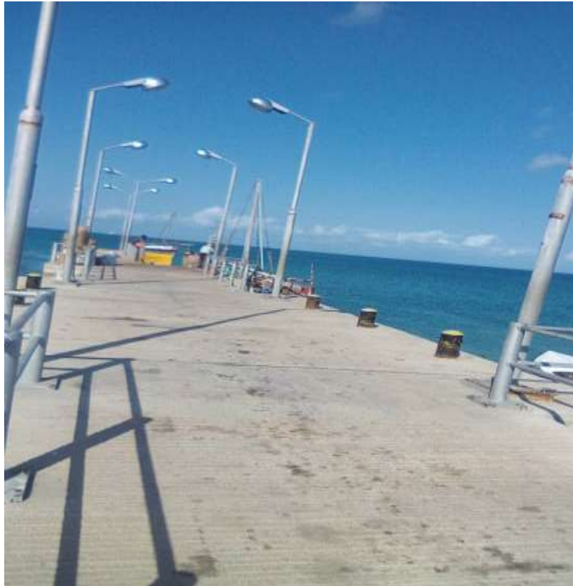
Figure 16: The operating Songosongo jetty rehabilitated by Songas Songosongo island Tanzania 2018.
