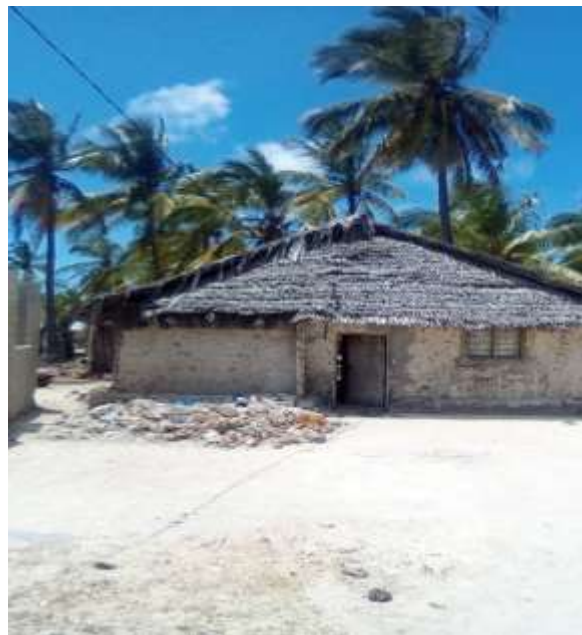
Figure 15: One of the electrified houses in Songosongo village Tanzania 2018.
