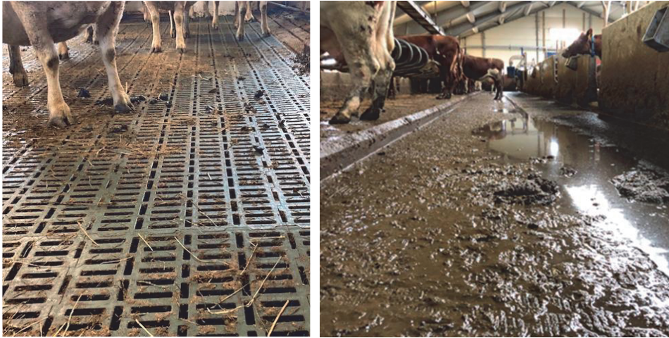
Figure 8. Sheep stall with plastic mesh flooring (left) and dairy freestall with closed flooring (right). Photo: Marit Smistad
