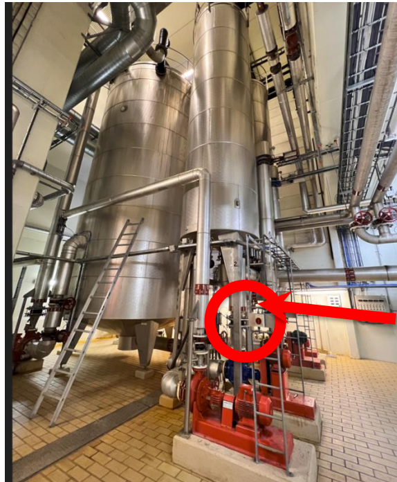
Figure 12: Buffer storage where the raw sludge was taken.
