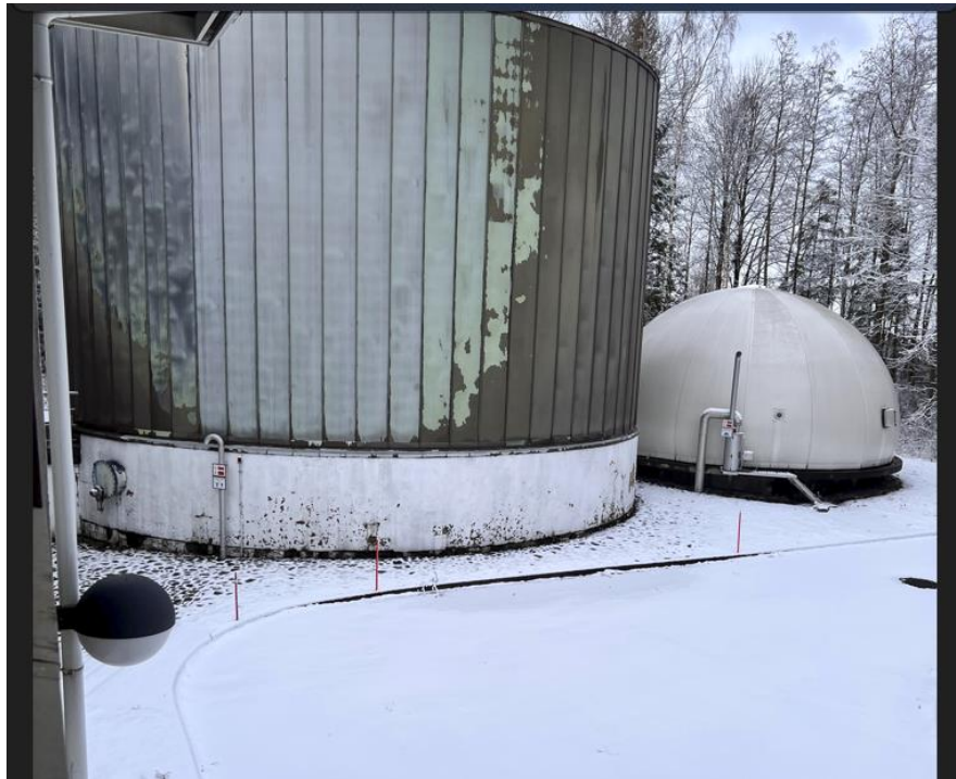
Figure 22: Anaerobic and gas reactor from outside.
