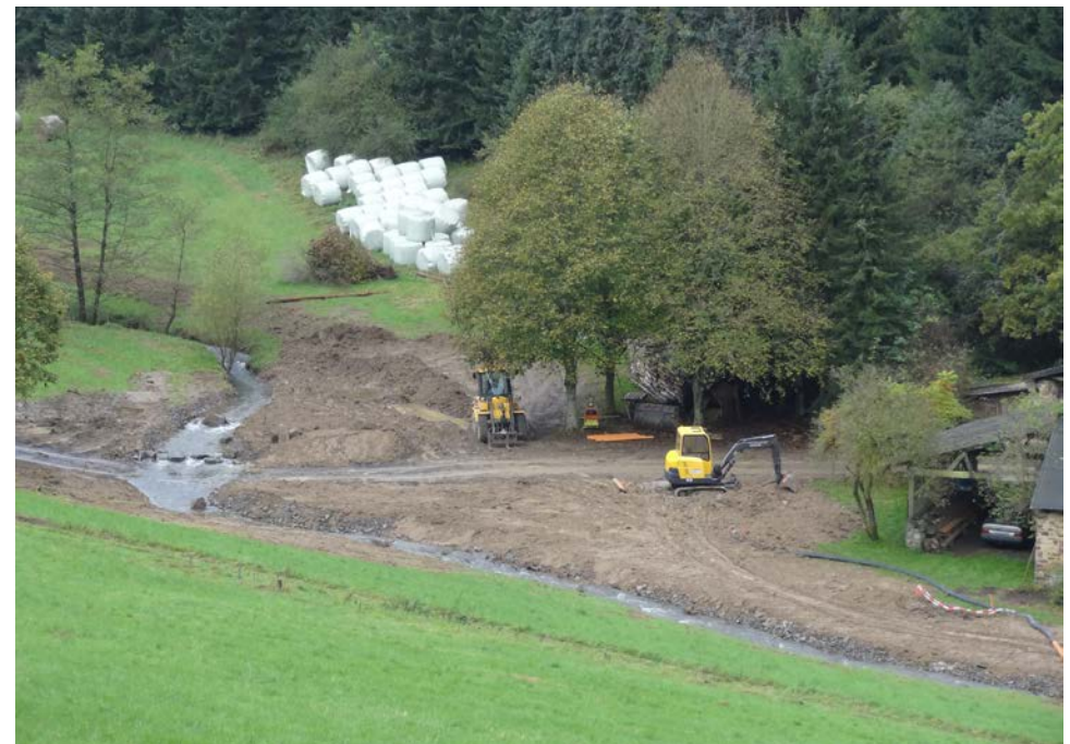
Nature-based solutions: reopening of piped streams at Kottenborner Mühle (Möller, 2022)
