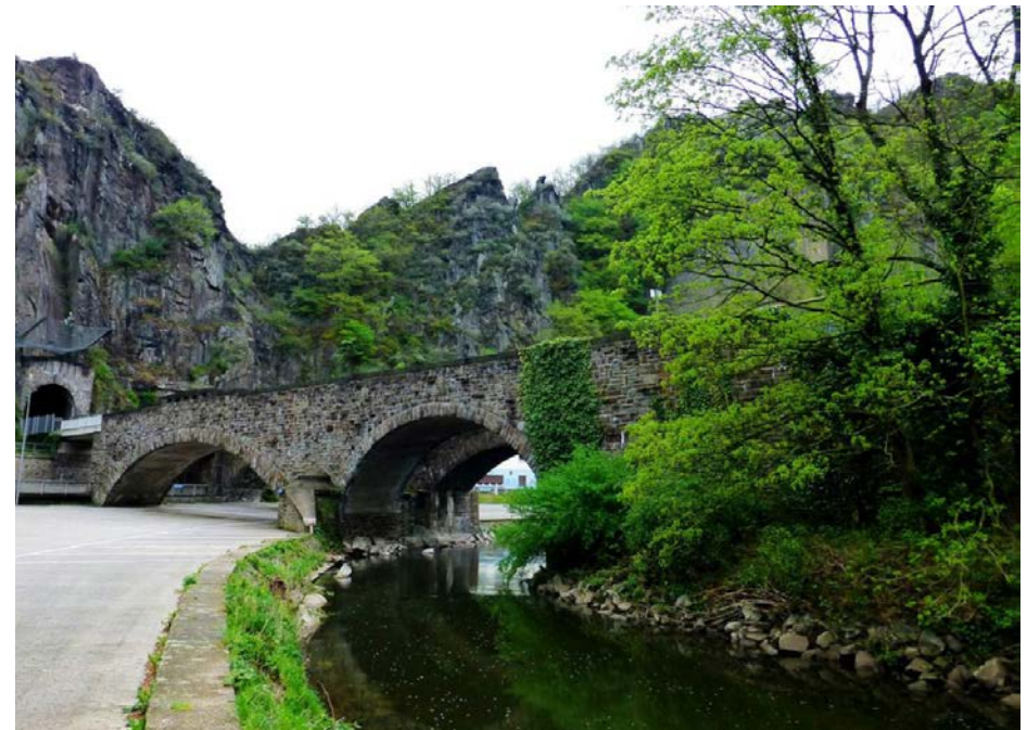
Railway bridge, Altenahr (Delminho, 2021)
