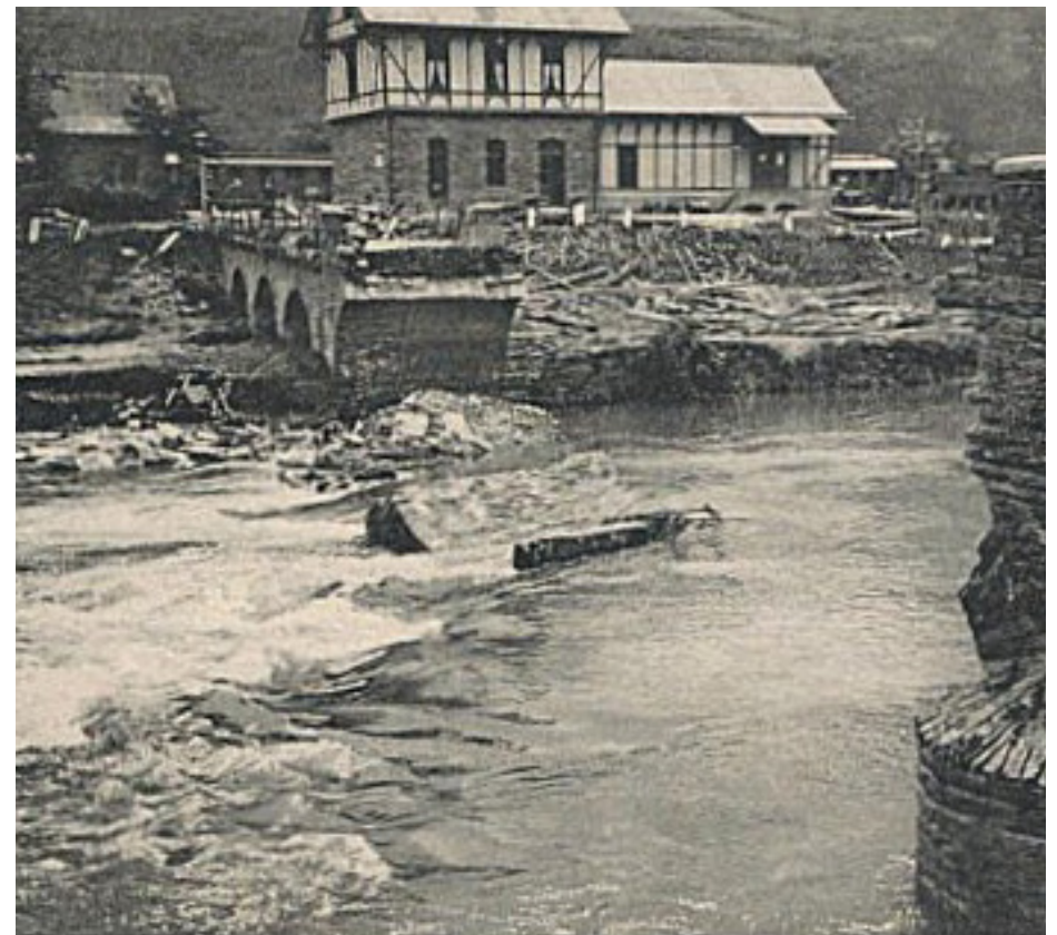
1910 flood, Mayschoss (Sinne, 2022)
