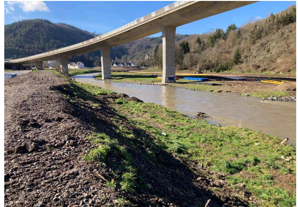
Railway embankment, Altenburg
