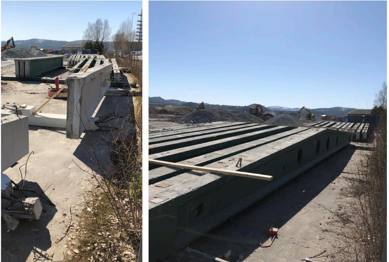
Figure 38 - Concrete beams (left) and ST-elements (right) extracted from demolition project in Namsos. Photo credit: Jon Aunet (author)
