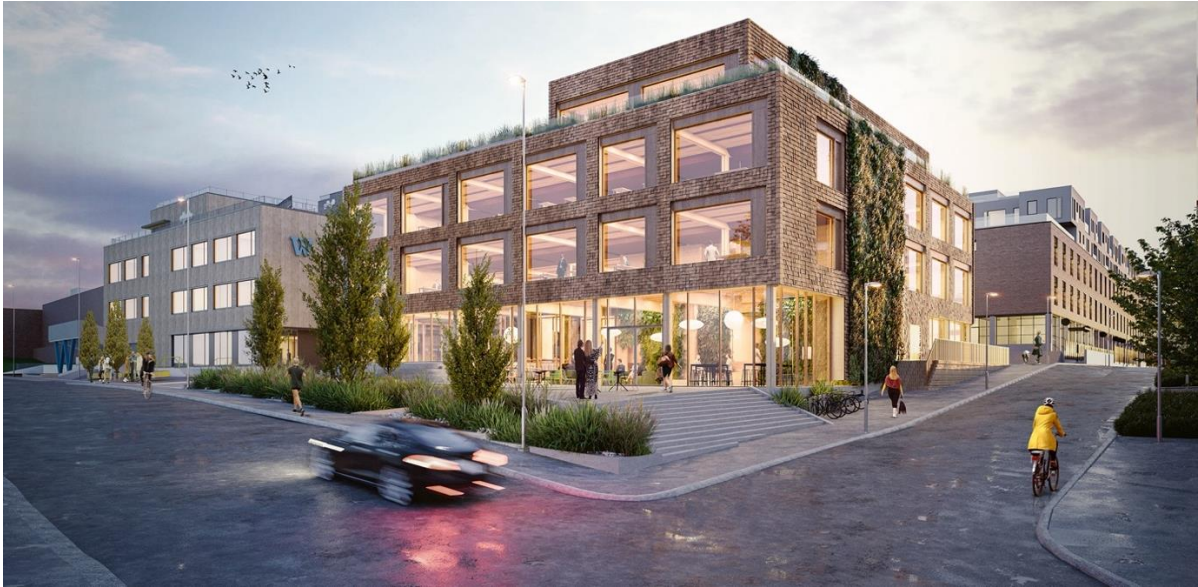
Figure 16 – Reusable commercial building in CLT and glulam (OsloTre, 2021).
