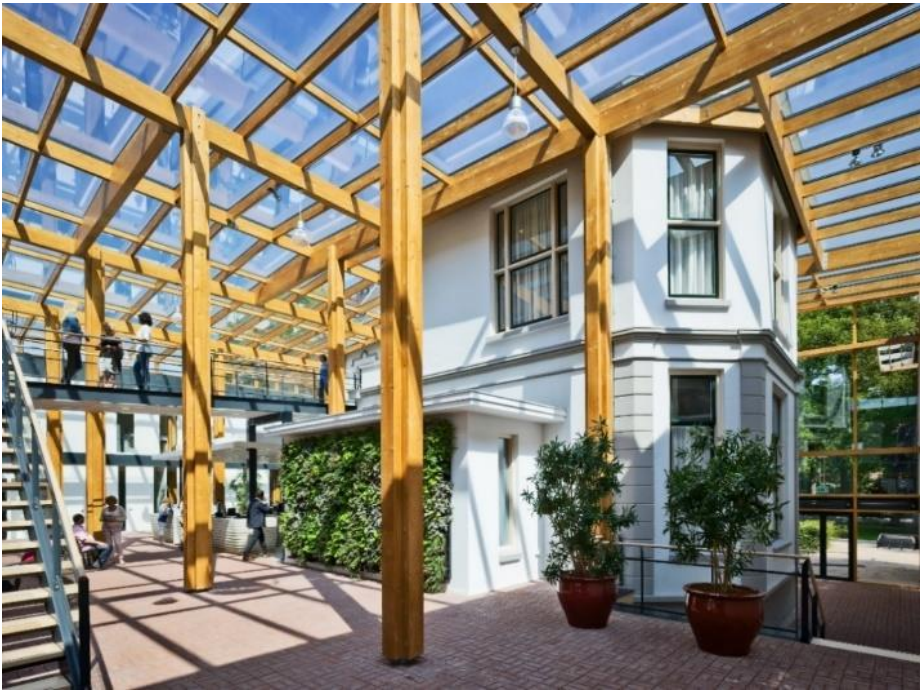
Figure 25 - Dismountable timber beams and columns in Brummen Town Hall (courtesy of Petra Applhof, RAU Architects)
