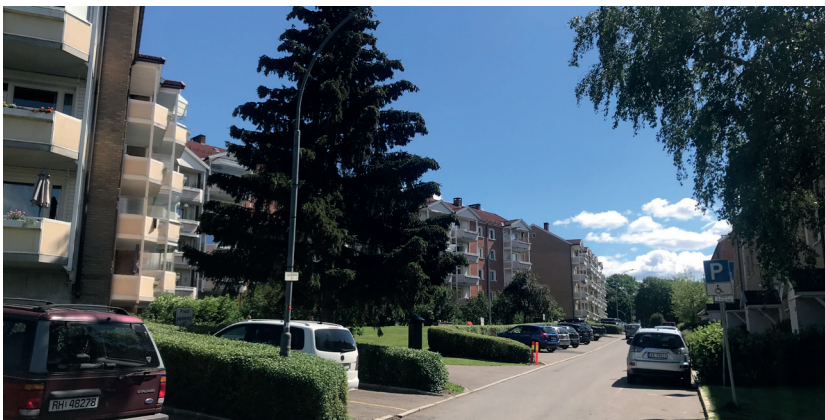
Figure 15 Relation between building and street – Lillebergveien Valle
