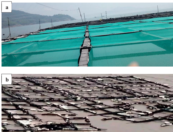
Figure 5. Traditional sea cages (a) Before typhoon; (b) After typhoon
