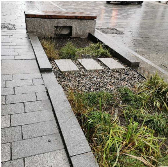
Photo 1. Example of Sustainable Urban Drainage System in Oslo. Photo: Michelle G. Johansen, 2020.
