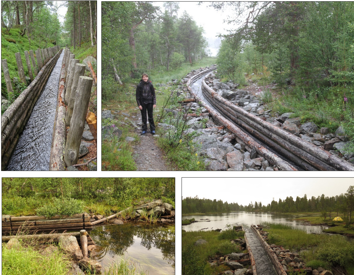
Timber flumes between Femunden and Feragen in Norway, connecting the Klarälven and Glomma watersheds. Photos: Eva B. Thorstad (upper left, lower left and right) and Odd Terje Sandlund (upper right).
