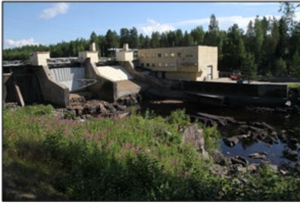
Lutufallet power station, which is the most downstream of the two power stations in Trysilelva in Norway. Photos: Odd Terje Sandlund.
