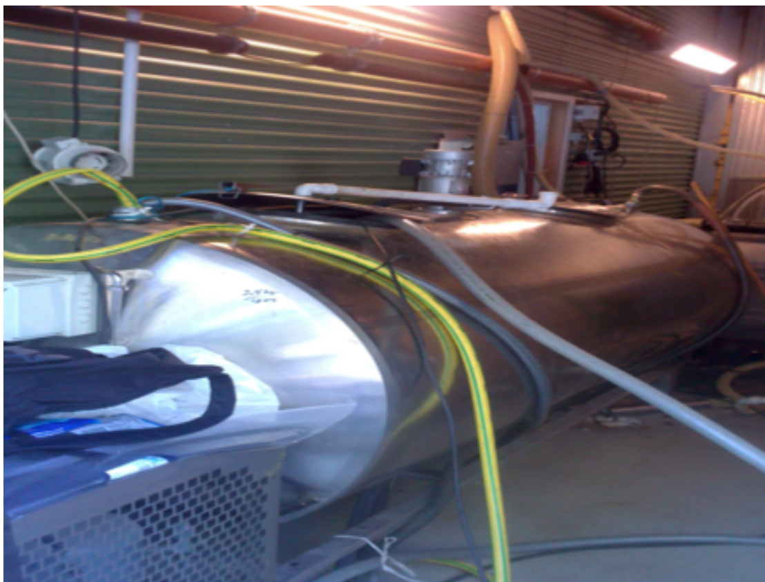
Figure 12.12: Greywater tank (Source: the author)
