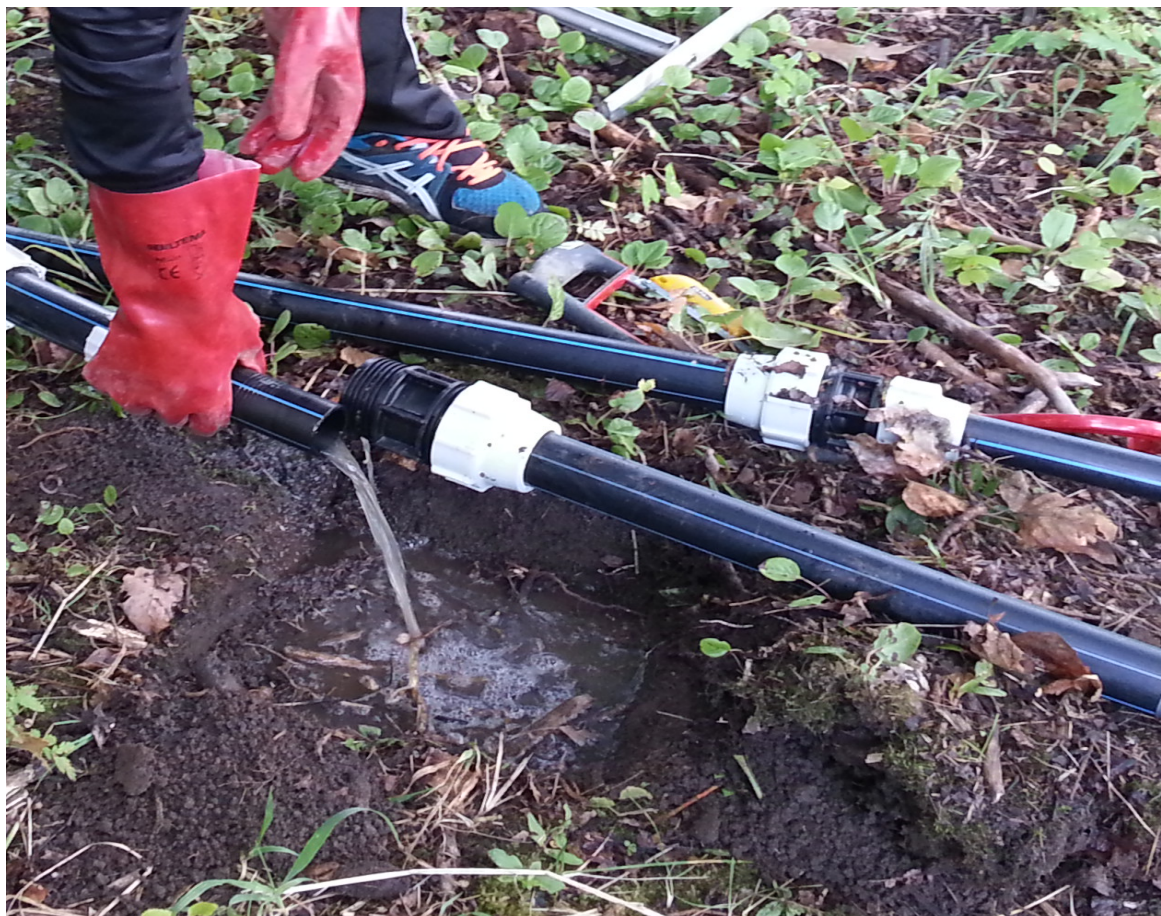
Figure 13.2: Testing segment check for 40 mm and 63 mm pipes (Source: the author)
