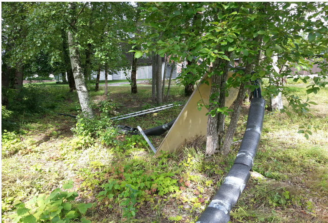
Figure 12.5: Slope for 40 mm and 50 mm SDR11 PE pipes (Source: the author)
