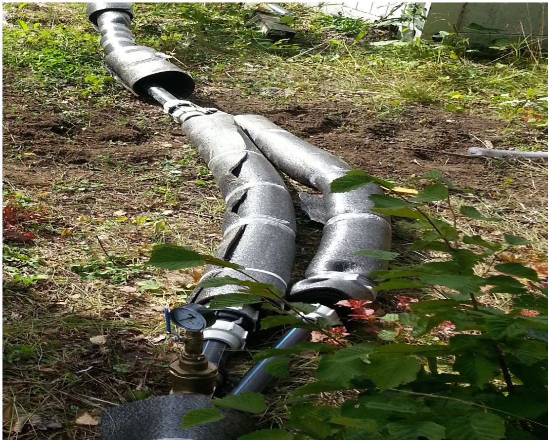
Figure 13.1: Checking sections on the 40 mm and 63 mm pipes (Source: the author)
