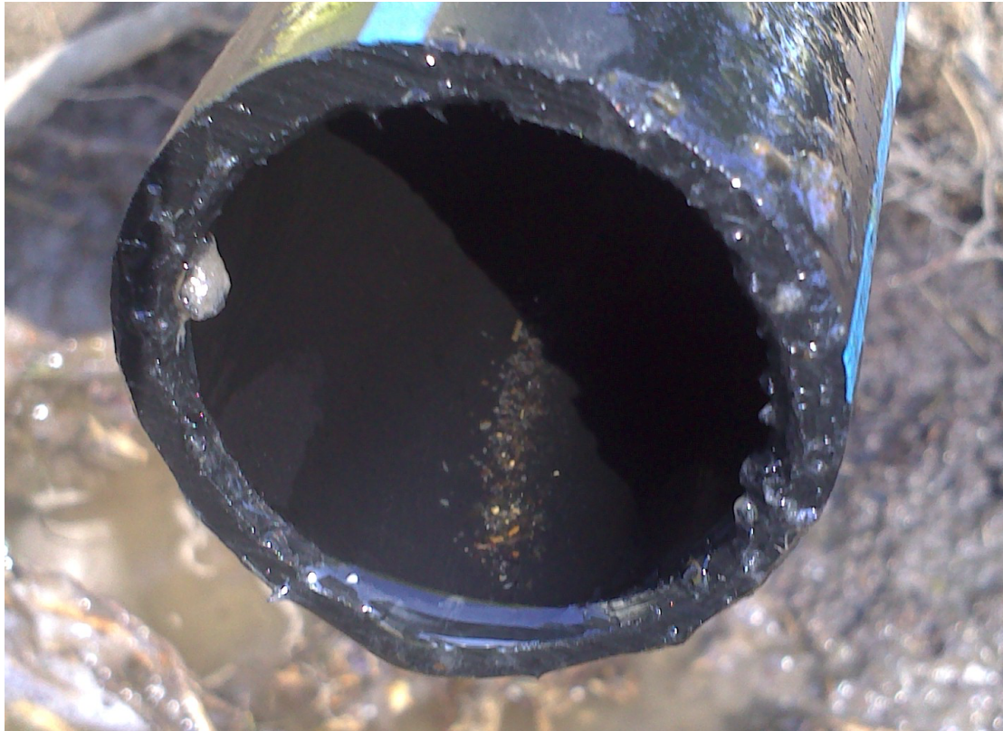
Figure 13.4: Opening of SDR11 PE 40 mm pipe (Source: the author)
