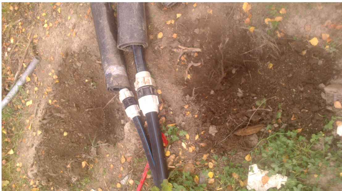
Figure 13.3: Finished check for 40 mm and 63 mm (Source: the author)
