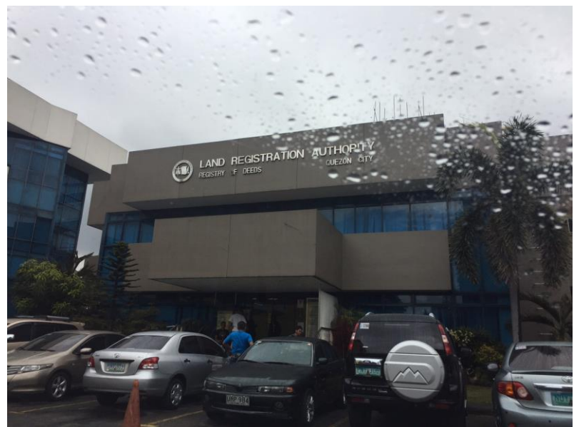
Photo 5- Land Registration Authority in Quezon City, Manila
