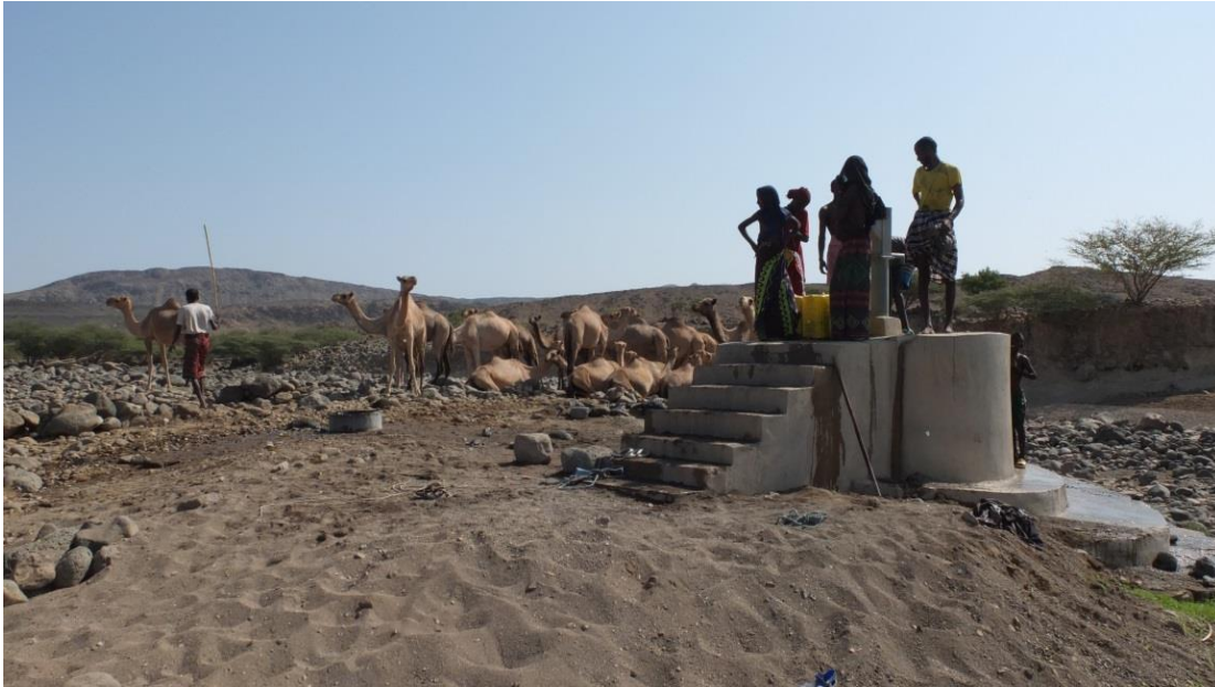
Figure 9: Cement boja . Community members of Serdo town fetching water from the cement boja that was constructed by the government (Photo: Siri Eggset, 2014).
