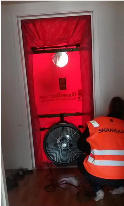
FIGUR 3-5: MONTERT BLOWER DOOR-VIFTE.
