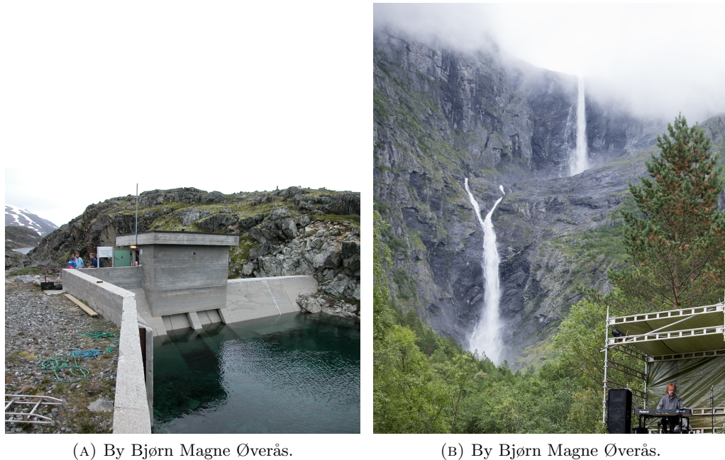
FIGURE 4.3: (a) The dam which regulates water flow from the lake Fossafjellvatn into the Mardøla river, which leads to Mardalsfossen waterfall. (b) Mardalsfossen under the Eikesdal town festival concert by Henning Sommero and John Pål Inderberg on the 9th of August 2014. The water flow was estimated to be around 2.5 \text{ m}^3/\text{s} - 3.0 \text{ m}^3/\text{s} .
