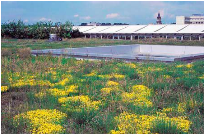
Figur 4: Semi-intensivt grønt tak (International Green Roof Association 2014).
