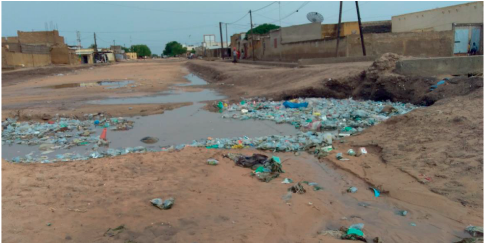
Figure 23. Empty plastic bags blocking a drain after heavy rains in Kaolack
