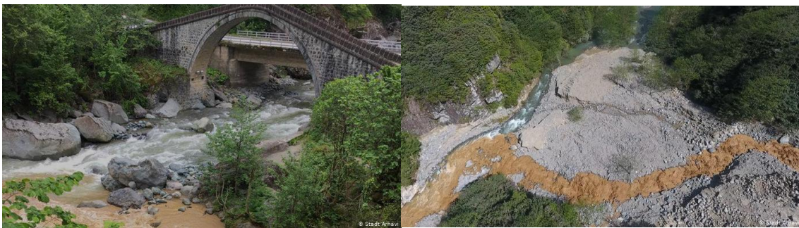
Figure 12: Downstream of Kamilet valley, after construction in 2020. Source: (Ocak, 2020)
