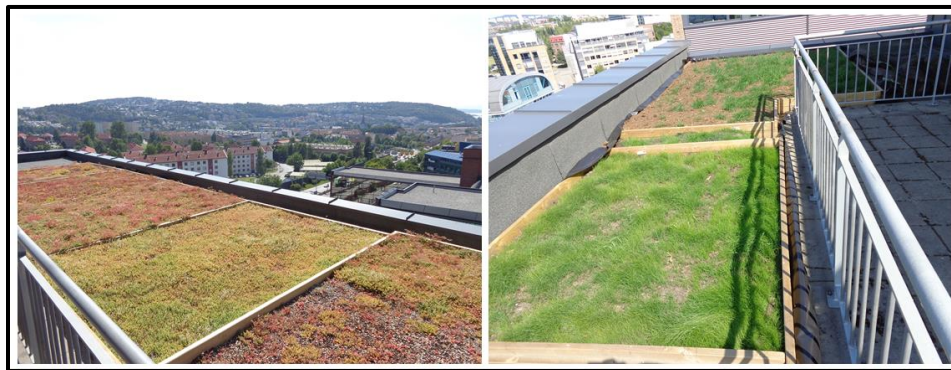
Figure 11 - Strømsveien 102 sedum roof (left) and turf roof (right)
