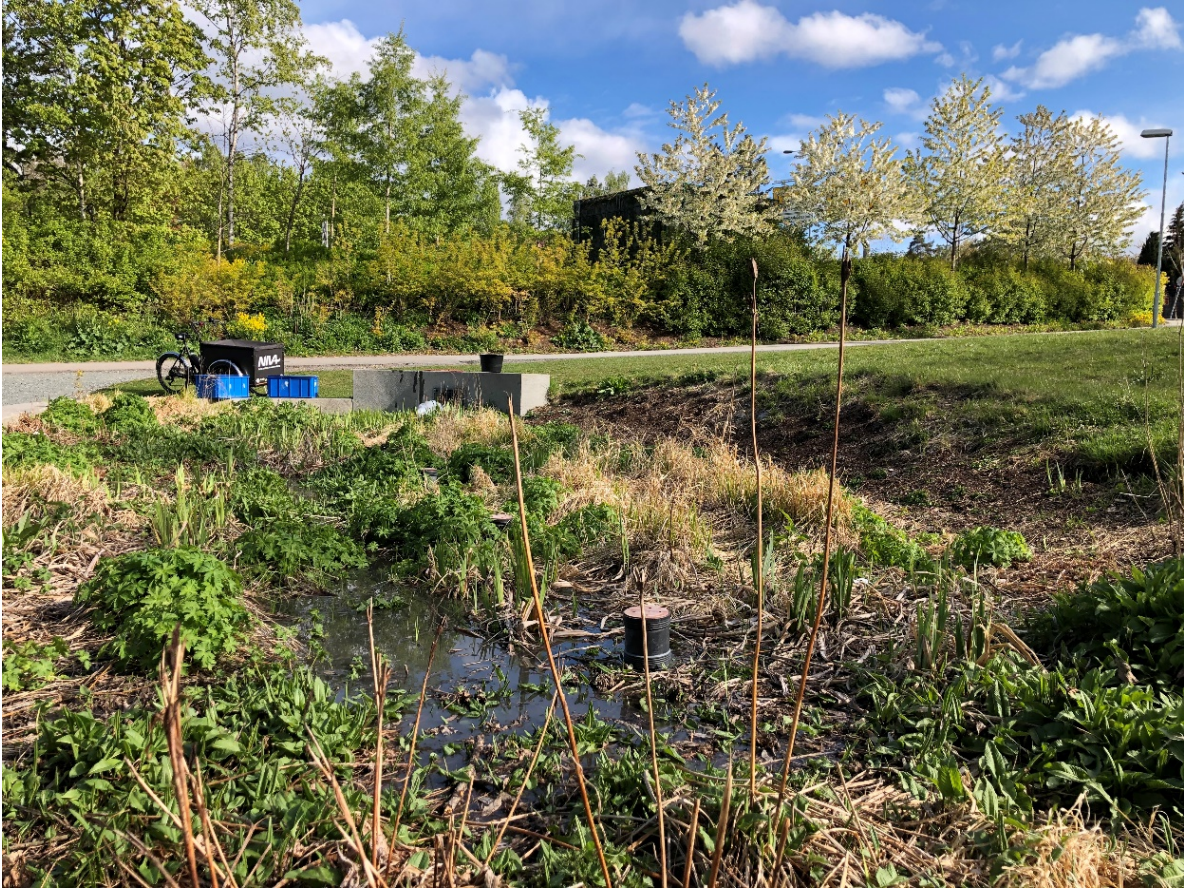
Figure 7. Example of a raingarden, applied as a second treatment step of tunnel wash water for the Smestad tunnel in Oslo, Norway (Photo: E. Rødland)
