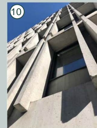
Figur 4.6. Fasadeelement i betong, Oslo MET.
