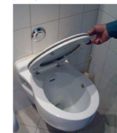
Figure 3: Vacuum toilet (source: Otterwasser)
