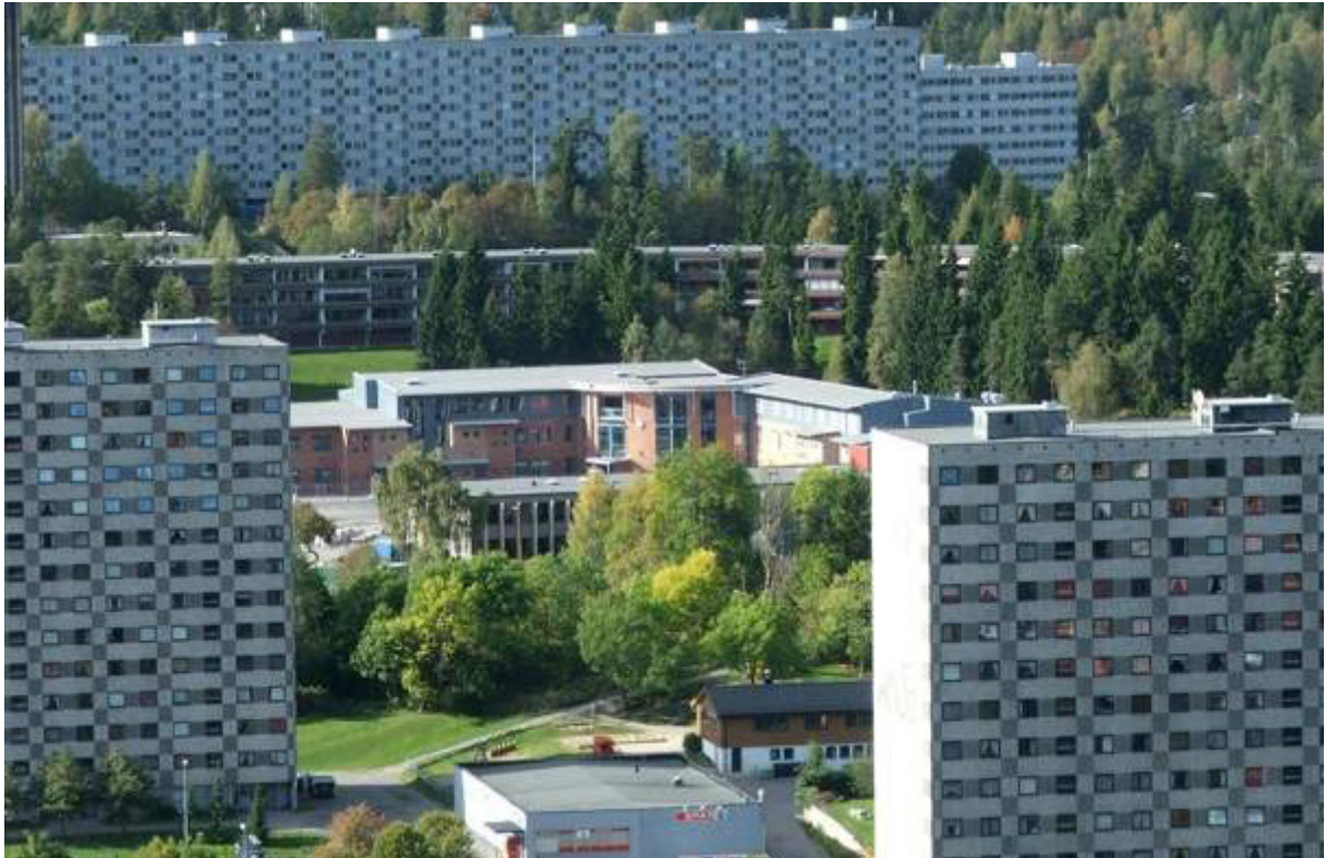
Fig. 4.7 Ammerud Elementary School behind apartment blocks
