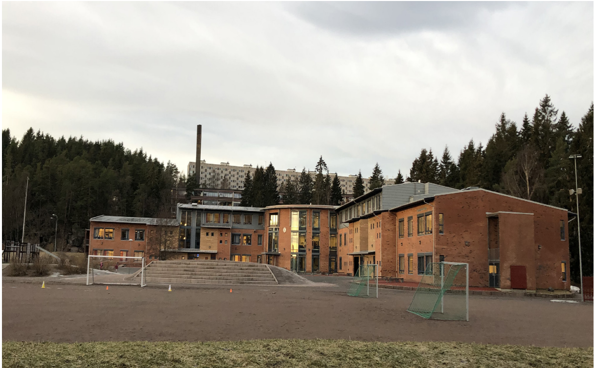
Fig. 4.6 Ammerud Elementary School
