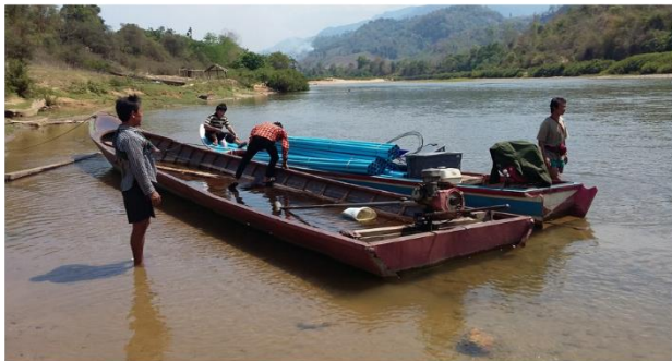
Picture 11: (top) Truck transporting PVC pipe. Picture 12: (bottom) Boats being loaded to transport cement and PVC pipe across the Moei river.
