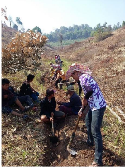
Picture 8: Villagers digging water pipeline
