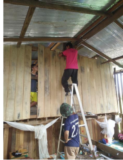
Picture 10: Villagers helping install AC electrical system
