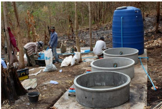
Picture 7: Construction of large bio-sand charcoal water filter in Kler Deh
