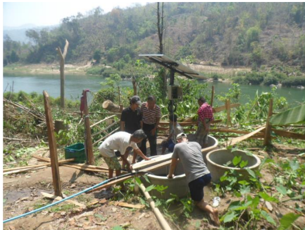
Picture 20: Installing solar pump at water source for Kler Deh school
