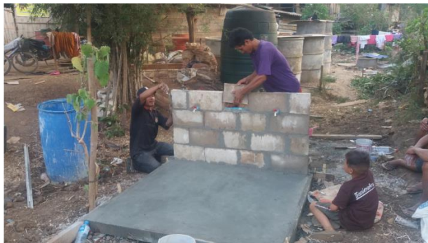
Picture 4: Construction of water access point in Hoi Nam Yen
