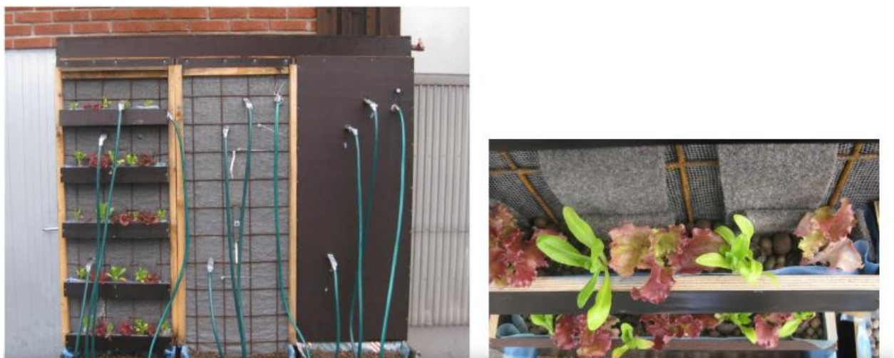
Completed filter wall (left) and details of planter shelves with felt strip irrigation system (right) (Svete, 2012).
