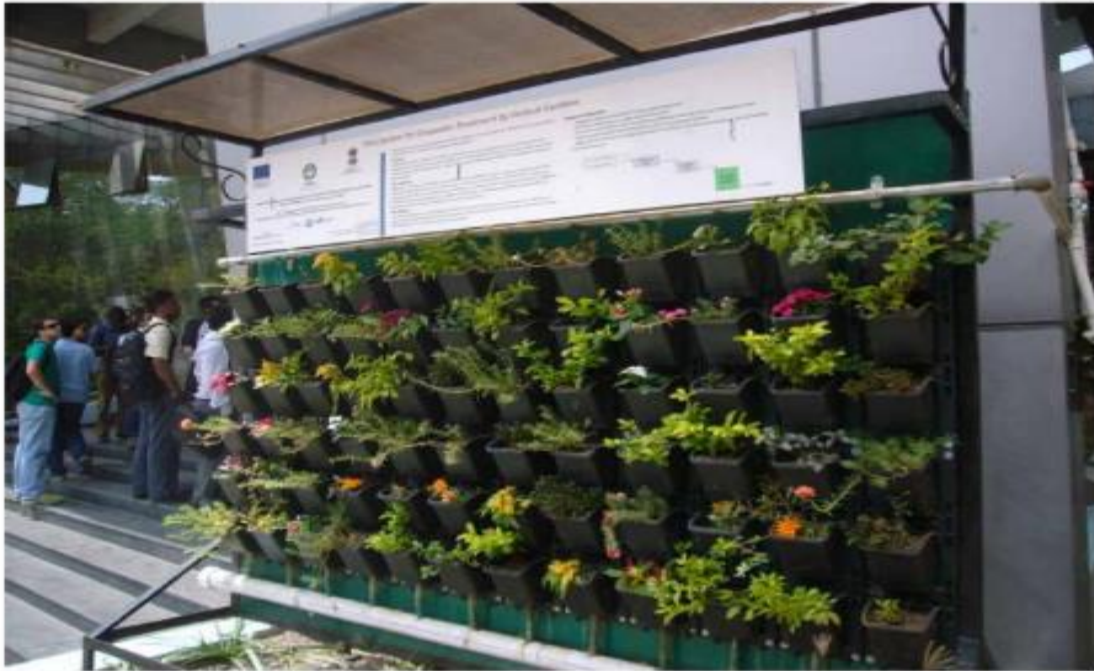
Figure 14. Green wall for greywater treatment installed at the MPs Head Office in Pune, India (Masi et al., 2018).
