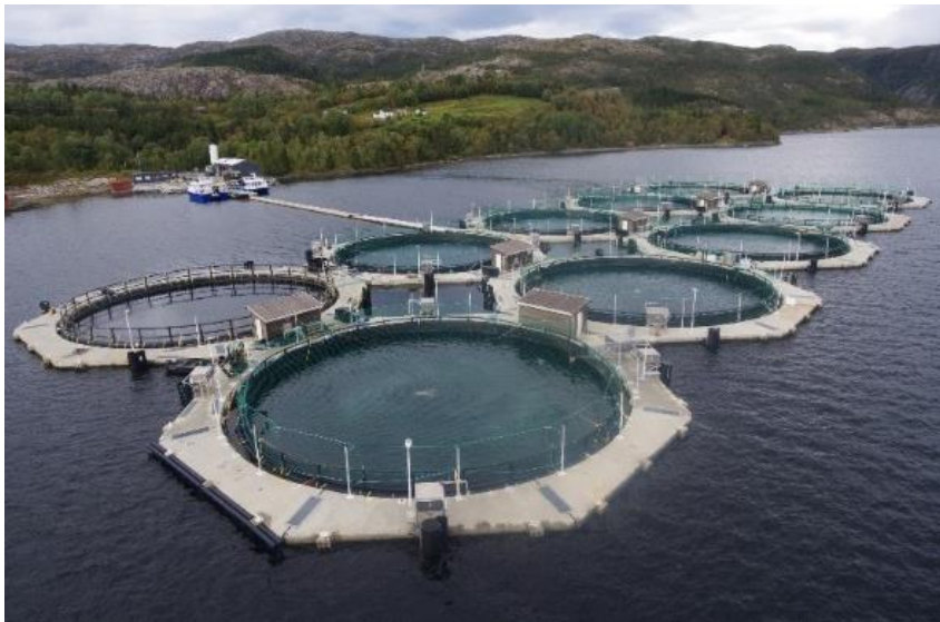
Figure 7. Above: Schematic illustration of a floating, tarpaulin cage (2870 m 3 ) with water intake from a 25 m depth, described in Papers I, II, III (Illustration: AkvaDesign AS). Below: Picture of a site with ten floating, tarpaulin cages (6000 m 3 ) of the same basic design, used for trials described in Paper II (Photo: AkvaFuture AS and Visual 360).
