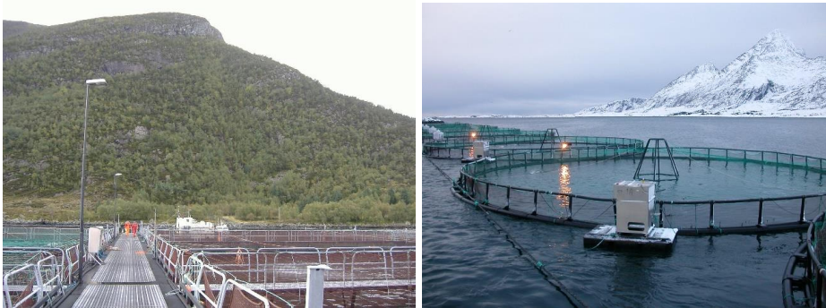
Figure 2. Examples of the new steel cages (left) and circular plastic cages (right) that dominated in Norwegian salmon and rainbow trout farms from 1990 (Photo: Arve Nilsen).
