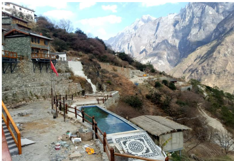
Figure 15 Construction of a tourist resort in Yachajiao village
