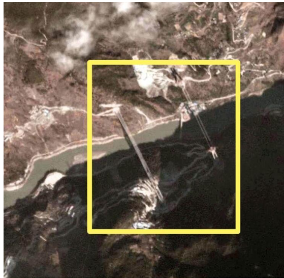
Figure 20 Aerial view of the two bridges in TLG From http://www.highestbridges.com/wiki/index.php?title=Jinshajiang_Railway_Bridge_Hutiaoxia
