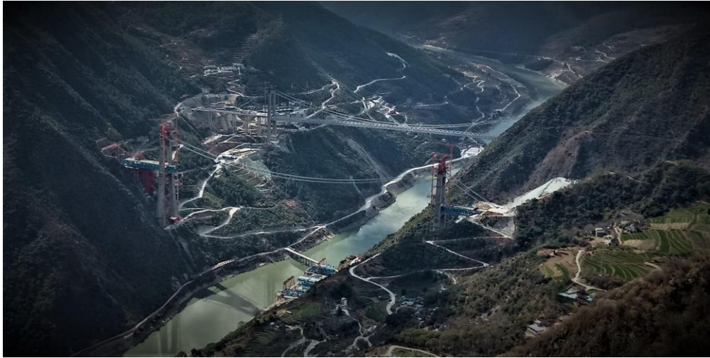
Figure 19 Construction of the Expressway bridge and Railway bridge over TLG
