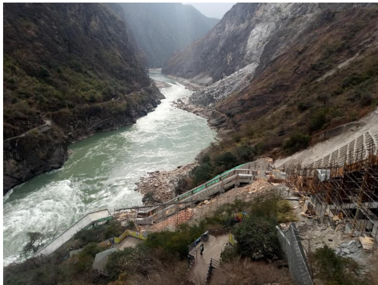
Figure 17 Elevator under construction in UGSA From: http://www.highestbridges.com/wiki/index.php?title=Jinshajiang_Railway_Bridge_Hutiaoxia
