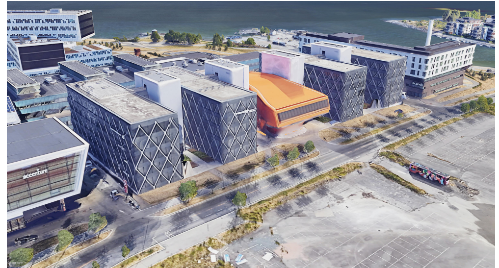
Figure 3.20: The Portal Building, Portalbygget (Google Earth, 2018).
