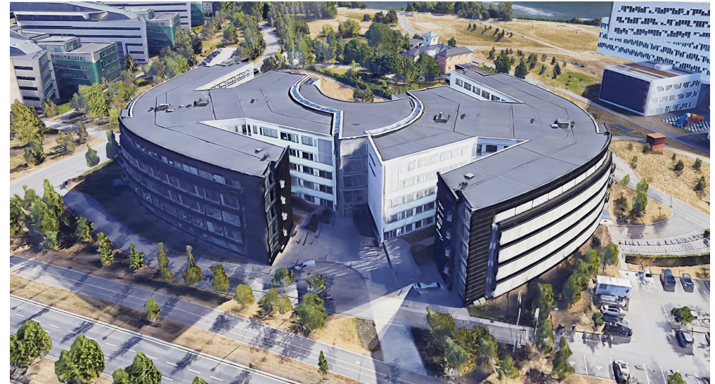
Figure 3.24: Fornebu Works (Google Earth, 2018).
