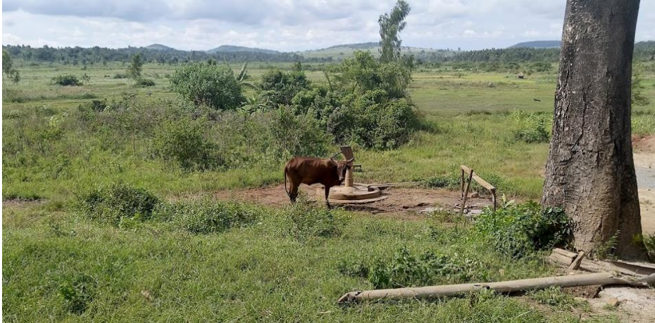
Figure 23: A cow was chained to the well to graze close to the well. This is highly problematic with regards to contamination risk due to the shallowness of the well.
