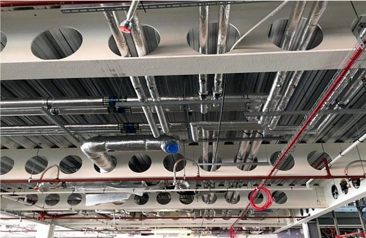
Figure 1 Service integration through the web-opening (Cellbeam Ltd, 2019)
