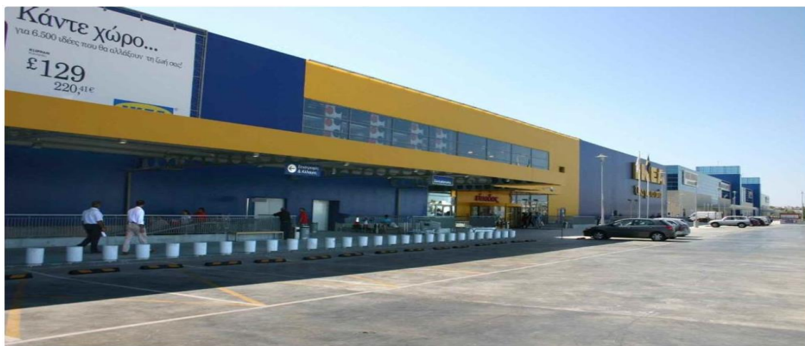
Figure 5 IKEA commercial center (Constructalia, 2007)
