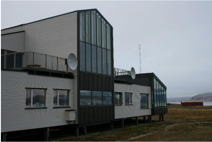
Figure 14. Picture showing the transmitting and receiving antennas mounted on the balcony on Kings Bay's service building in Ny-Ålesund in 2009. Photograph courtesy of ISPAS AS.
