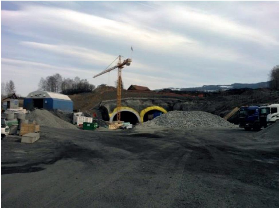
Figure 5: Tunnel construction at Gran.
