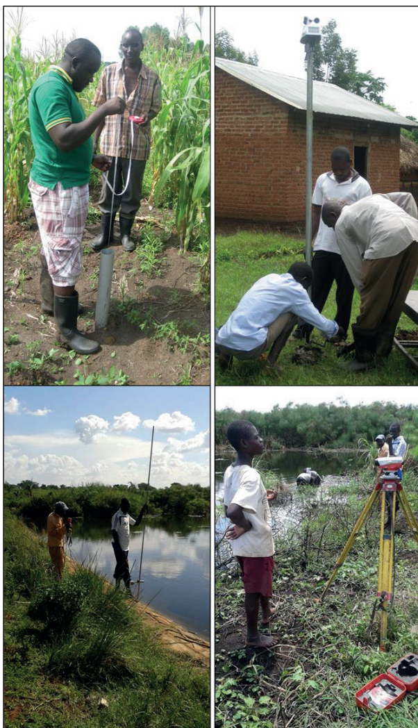
Figure 5: Clockwise from top left: borehole monitoring, setting up weather station, installation of water gauges at wetland in lets and outlets, discharge measurements
