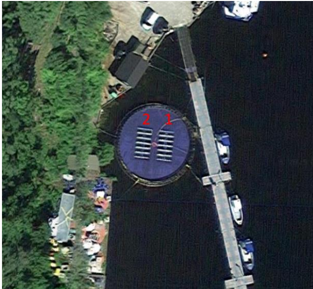
Figure 19: Picture of the system at Skaftå as seen from above. The number one and two marks the string numbers [30].
