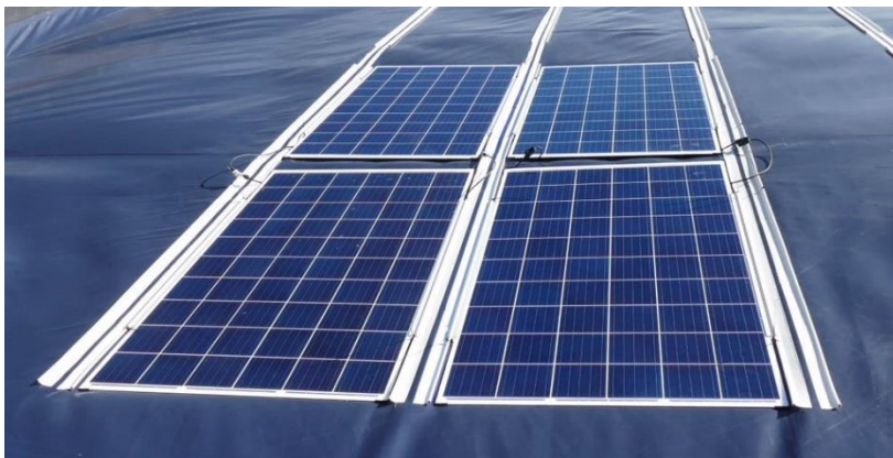
Figure 14: Ocean suns floating PV technology [29].
