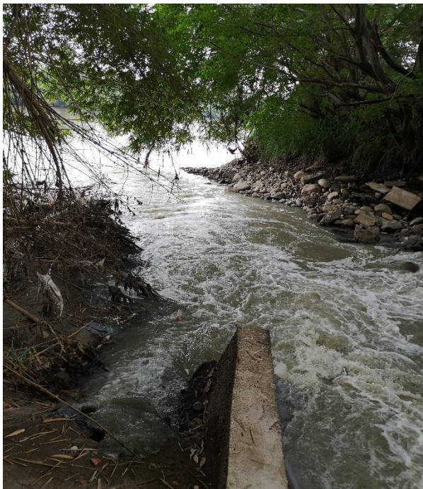
Figure 4. Puente Santander North point
