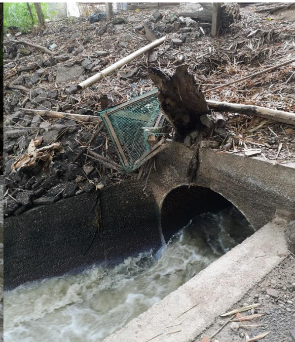
Figure 5. Puente Santander South point
