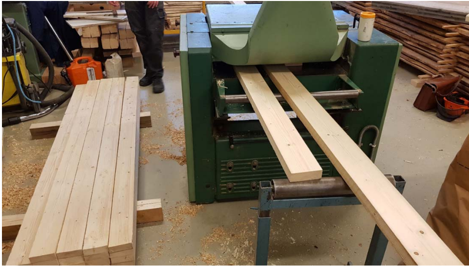
Figure 15: Preparation of timber boards
