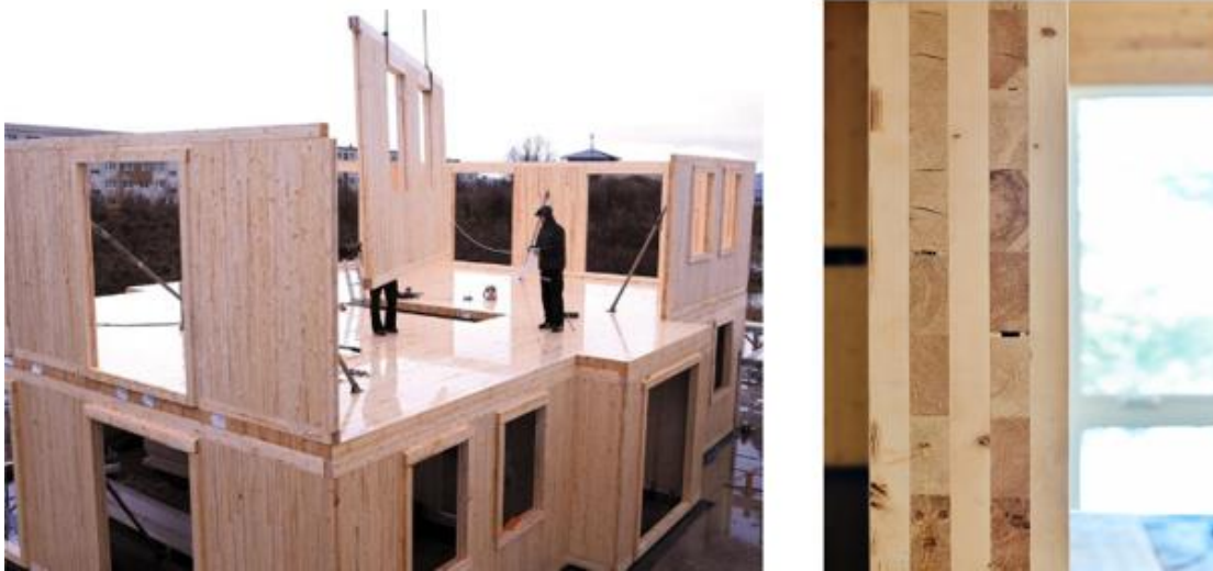
Figure 2-18: CLT wall construction (Companies; Franco, 20.May.2018)
