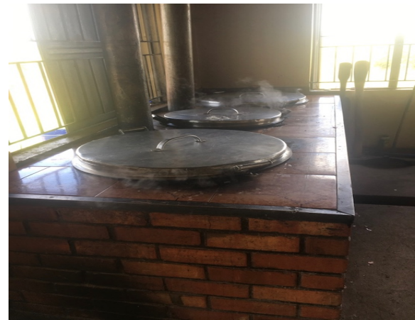
Figure 2.7 The stove inside the kitchen where the food is prepared
