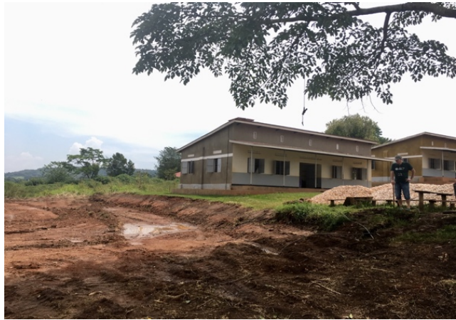
Figure 2.2 Construction site of the main hall and kitchen
