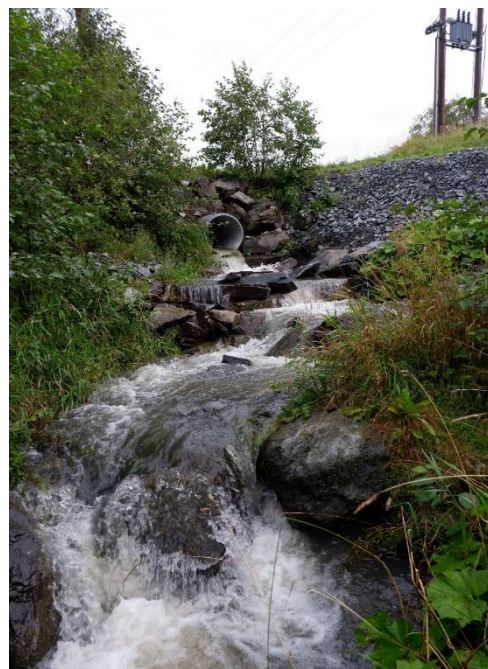
Figure 27: Culvert at the end of station 2 under road Vukuvegen in Follobekken.
