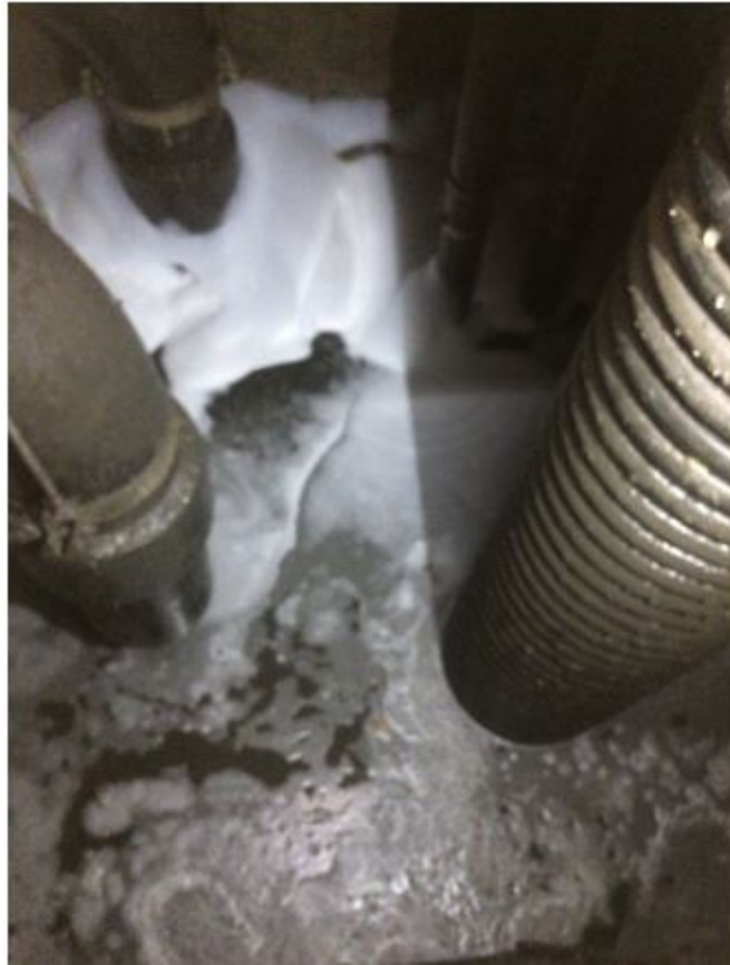
Figure 3.4: pumping chamber with foaming soap during tunnel wash. Photo: Ninni Bye.
