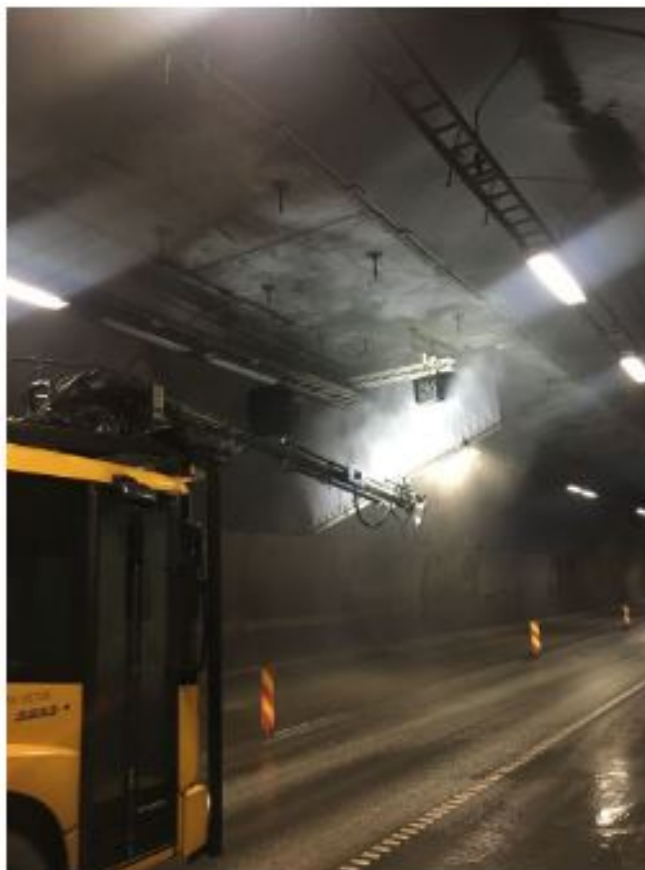
Figure 2.6: Tunnel wash. Photo: Jon Petter Johnsen.
