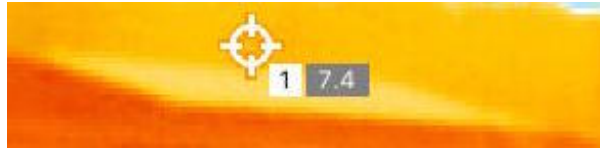
Figure C.4: Two thermal images of system 5, taken from different angles, indicating a constant temperature over the entire system. Note that the absolute temperatures shown in the images is wrong as temperature and emissivity references were not possible to set.
