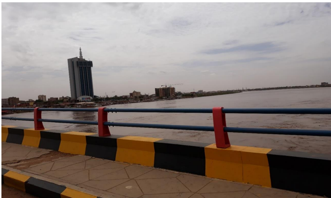
Figure (7) El-Manshia Bridge 33 connects El-Gerief East to Khartoum
