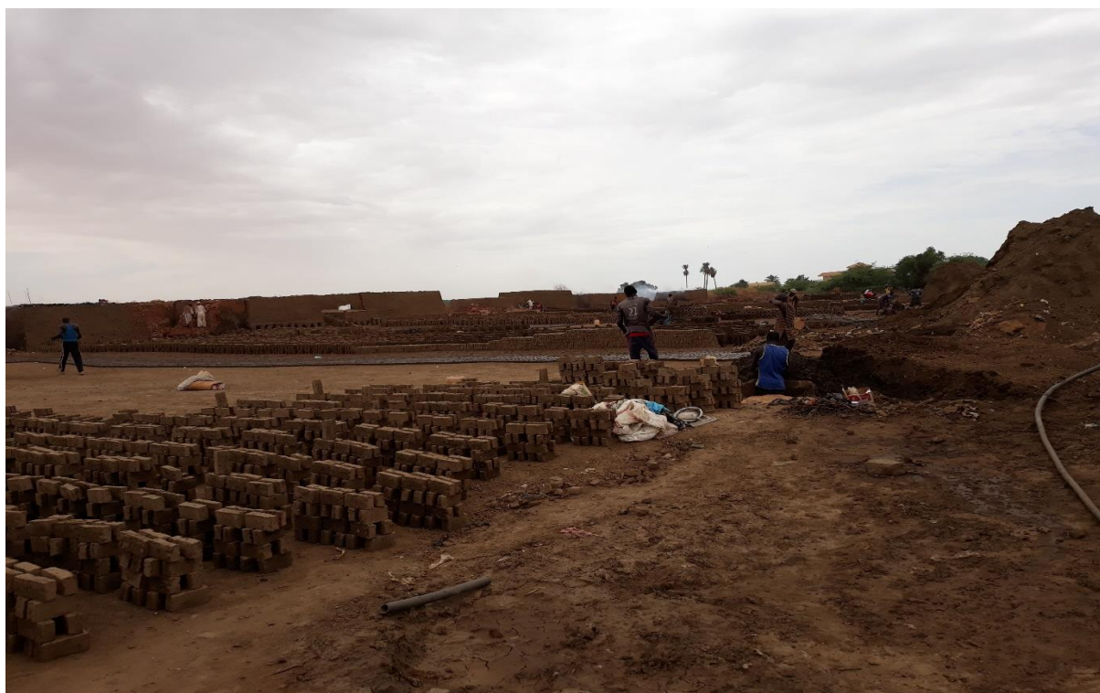
Figure (10) Photo shows the Kamāyin site in El-Gerief East
